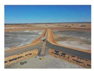
Scope The objective of the TSFE4 project was to provide tailings storage capacity for 30 months production with a 3.5m raise of Cell 3 to RL 271.1. The execution phase scope consists of mechanical works on tailings delivery and decant recovery systems, civil earthworks to construct the raise utilising in-situ tailings for working platform and local clay borrow materials for the raise; and installation of an internal tailings drainage system to improve tailings consolidation for future raises.
