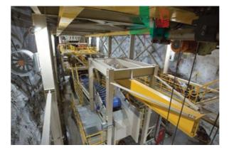
Scope Construction of a replacement underground mining primary crushing in an active underground mining environment. Work involved all civil, mechanical piping, and electrical instrumentation works to provide a fully functioning primary crushing system. The business-critical project was executed under continuous shift or roster cycles, successfully delivered on time and on budget without incident.
